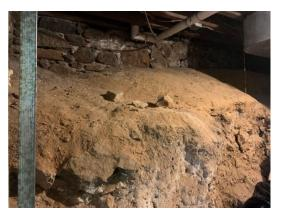
basement collapsed, causing stones and dirt to invade the building (image depicted to the right). This collapse has called into question the existing structural integrity of the building's foundation. 43. Mendham United Methodist is also concerned with preserving and repairing its bell tower. Passersby in front of the church can see the damage to the bell tower's siding (image depicted to the right). Given that the bell tower is a focal point of the building's historic architecture, it is
